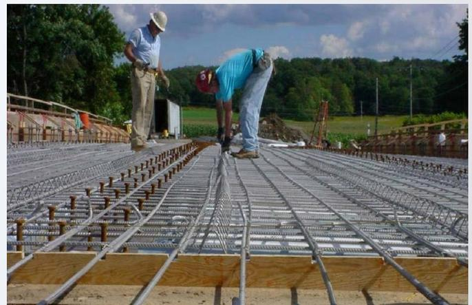
Installation of stainless steel rebar at the French Creek Bridge, Chautauqua Co., NY. (Photo Courtesy of Dunkirk Specialty Steel)
