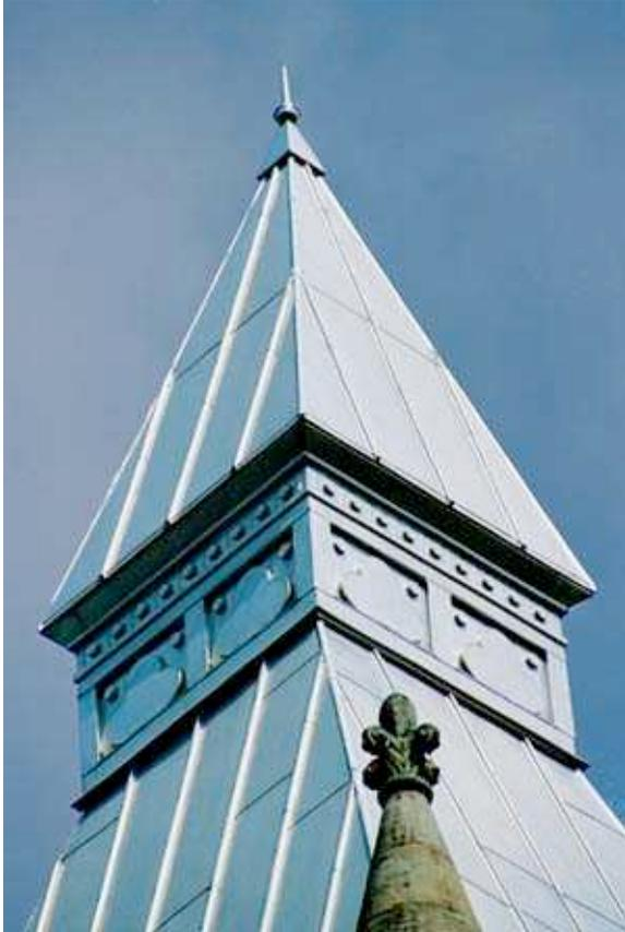
Figure 3: The Type 302 stainless steel roof on the Butler County Court House has provided about 80 years of trouble- and maintenance-free service. Photo credit: Catherine Houska, TMR Consulting
