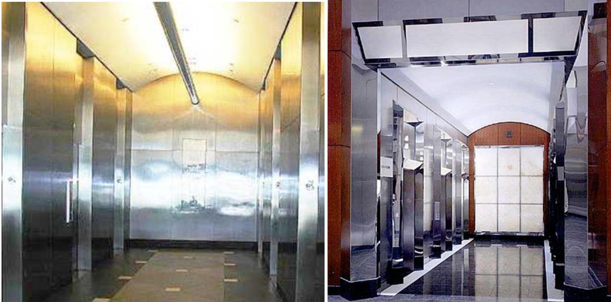
Figures 8 and 9: The stainless steel panels in the lobby of 525 William Penn Place in Pittsburgh had become dirty and scratched after about fifty years of use. During renovation of the lobby of 525 William Penn Place, the 50-year old stainless steel panels were removed, cleaned, refinished, and reused. (Photo credits: Catherine Houska, TMR Consulting and IKM Inc.)
