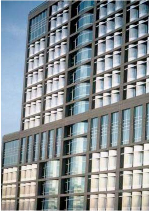
Figure 5: Stainless steel polished and perforated window screens on the Phoenix City Hall dramatically reduced air-conditioning costs and improved worker comfort. Photo courtesy of Allegheny Technologies.
