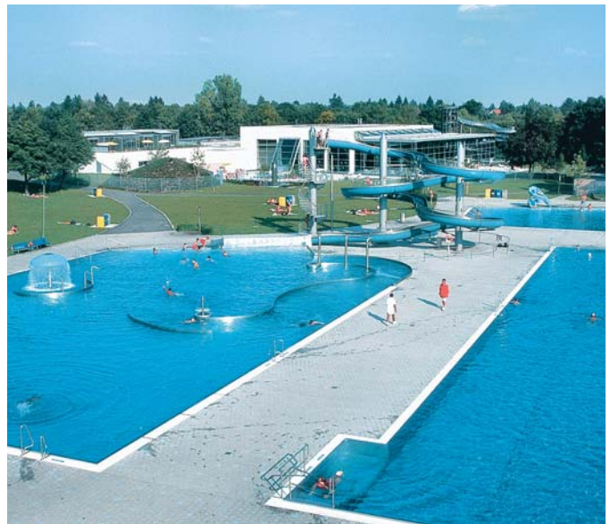
Figure 8: This swimming pool in Munich, Germany was relined with Type 316 stainless steel panels that were welded together. Photo courtesy of Martina Helzel
