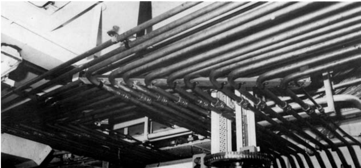
A multi-tube installation in 90/10 copper-nickel alloy for hydraulically operated controls for ESV "Iolair". (Yorkshire Imperial Alloys)
