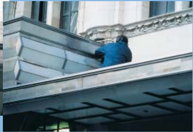
A worker hand-cleaning the canopy
