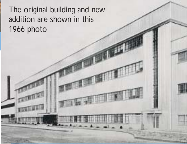
Courtesy of the American Iron and Steel Institute
