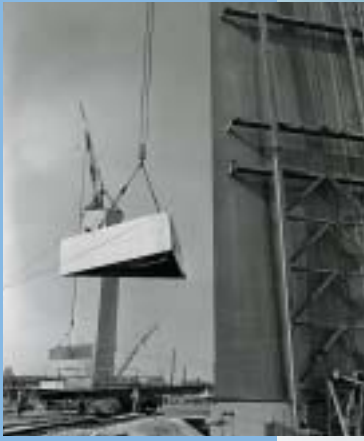
Construction of the Gateway Arch
