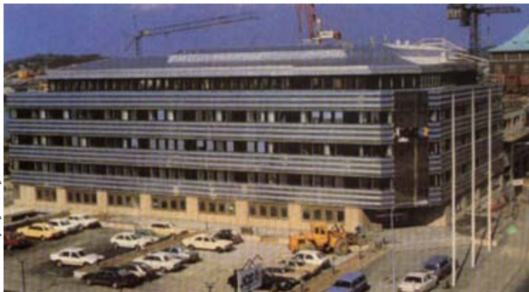
Courtesy of Rostfria Tak AB, Sweden
