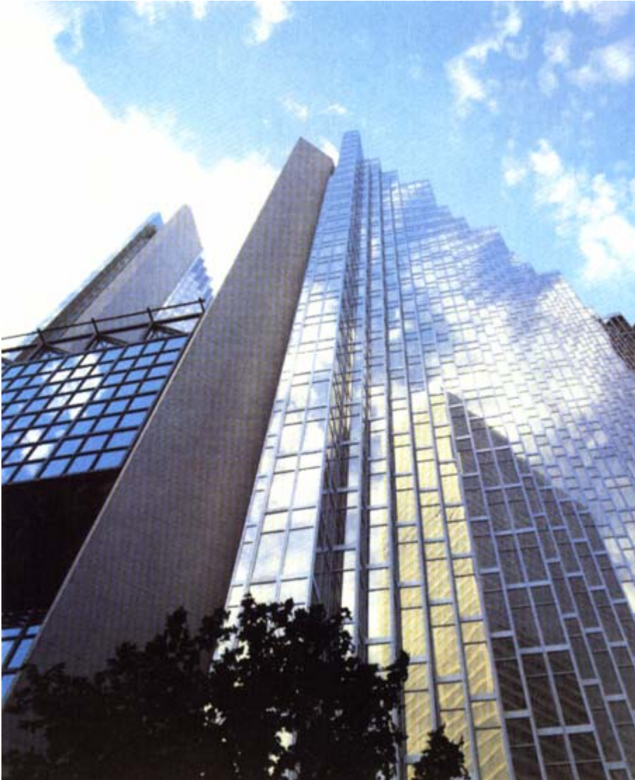
Royal Bank Plaza, Toronto, Canada. The mullions and spandrels for the curtain wall utilise nickel stainless steel AISI Type 304 in thicknesses of 0.78 mm and 1.57 mm respectively.
