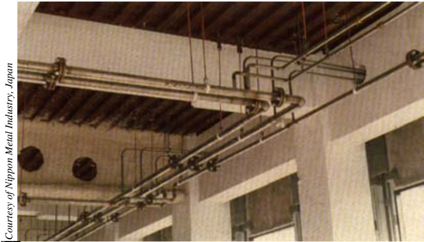
Water supply tubing in nickel stainless steel.
