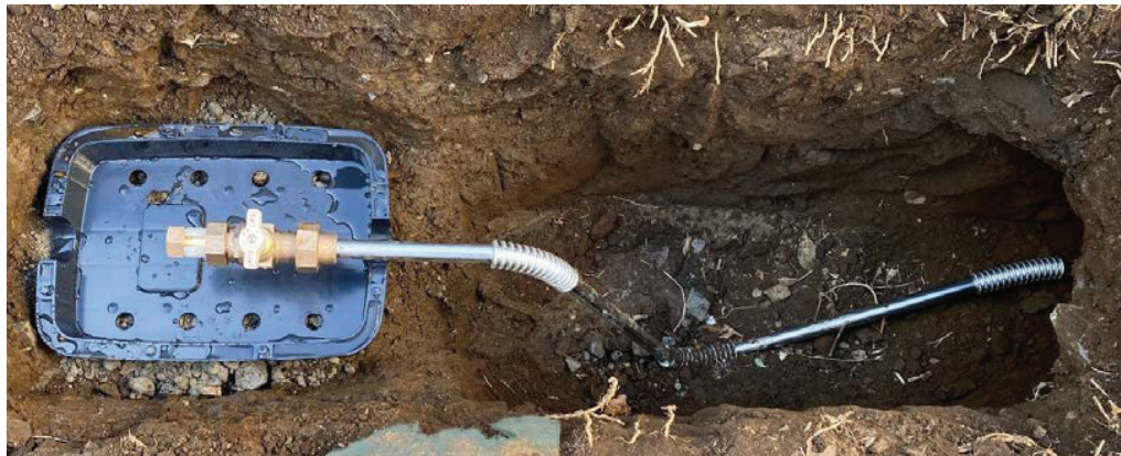
Image 2: Installation of SPCT in Tokyo / photo Nicole KINSMAN.
