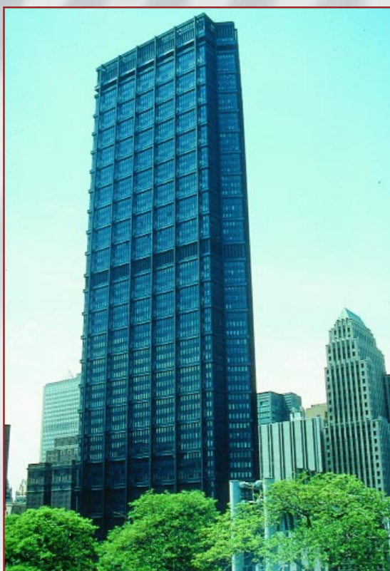
The USX Tower has a CORTEN exterior (a weathering steel exterior) and was completed in 1971. The CORTEN was allowed to weather naturally but was eventually painted because the rust was staining nearby buildings. Architect: Harrison and Abramovitz.
