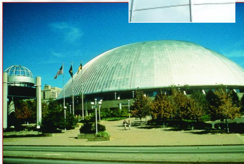
The Pittsburgh Mellon Arena had the largest dome in the world and largest retractable roof when it was completed in 1961. The roof is Type 304 stainless steel. Architect: Dahlen K. Ritchey.
