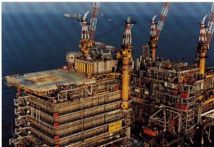
Stainless steel cladding, as used for this British Gas platform in Morecambe Bay, ensures long trouble-free life, minimum maintenance and outstanding resistance to fire.
