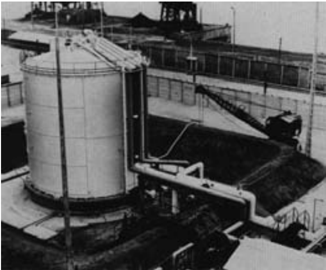
Figure D LNG tank of 9Ni steel built for Gaz de France in Nantes, France – 1960. Courtesy GDF
