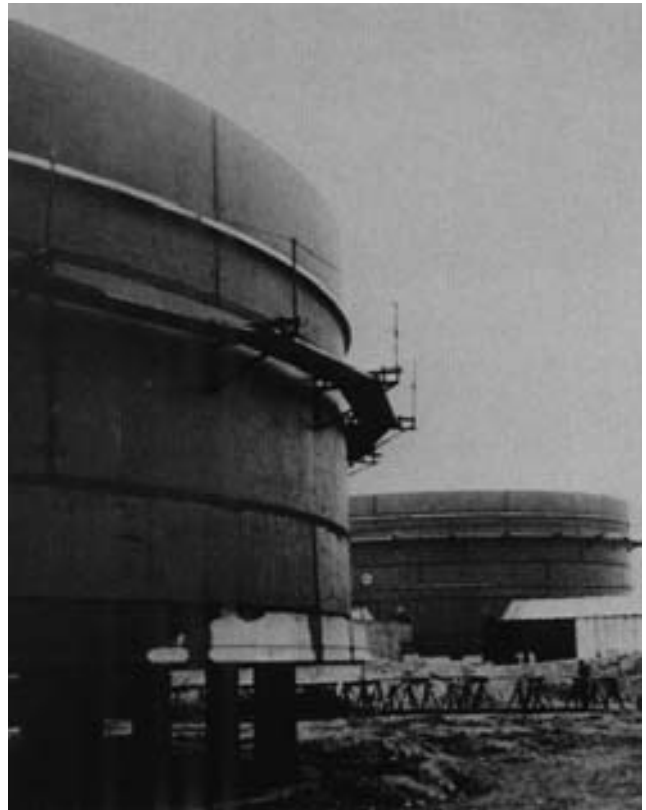
Figure E Two of three 9Ni tanks at Le Havre built to receive LNG from Algeria. Courtesy GDF
