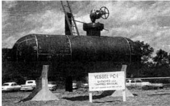
H1 – Test pressure vessel of quenched and tempered 9Ni steel not stress-relieved after welding
