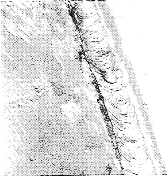
Figure 9 Corrosion at the toe of a vertical weld, probably from residual slag.
