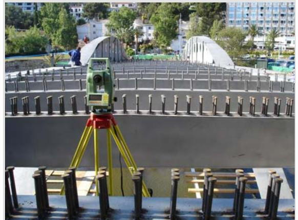
Figure 12: Shear connectors on transverse beams
