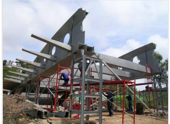
Figure 11: Temporary supports for the main structure
