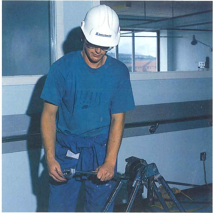
Stainless steel tubing is bent in the usual way
