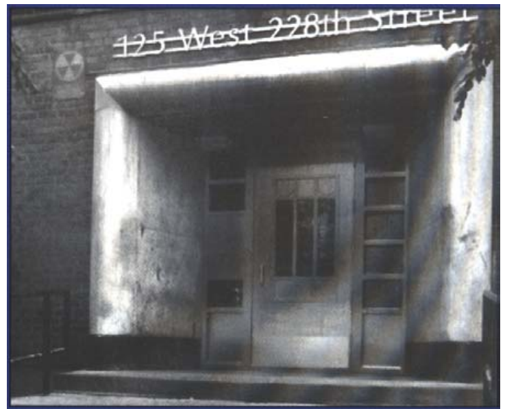
Type 316, all-stainless steel doors on the New York City Housing Authority's Marble Hill Houses.
