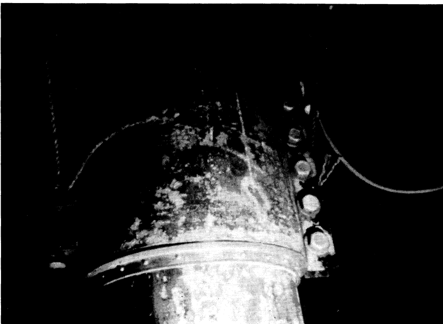
Offshore drilling platform using alloy K-500 bolts in riser clamps.
