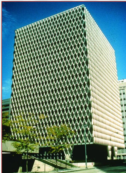
The United States Steel Worker's Building (formerly the IBM Building) was completed in 1963. It has Type 304 stainless steel cladding on the steel lattice trusses and anodized aluminum panels under the windows. Architect: Curtis & Davis.
