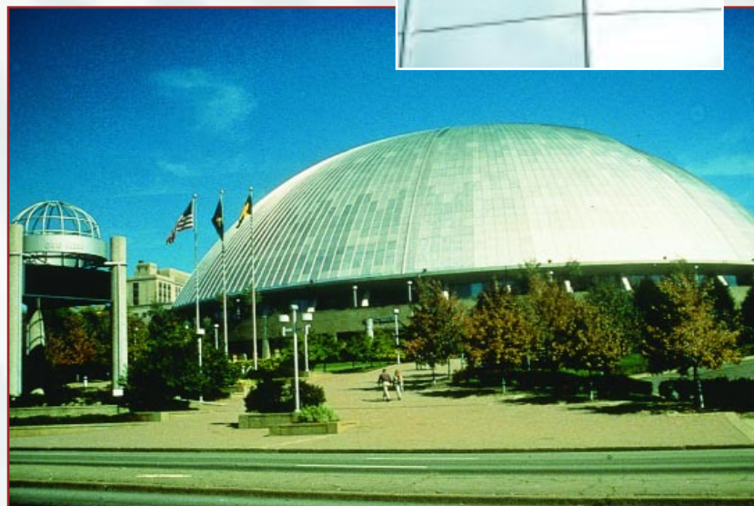
The Pittsburgh Mellon Arena had the largest dome in the world and largest retractable roof when it was completed in 1961. The roof is Type 304 stainless steel. Architect: Dahlen K. Ritchey.
