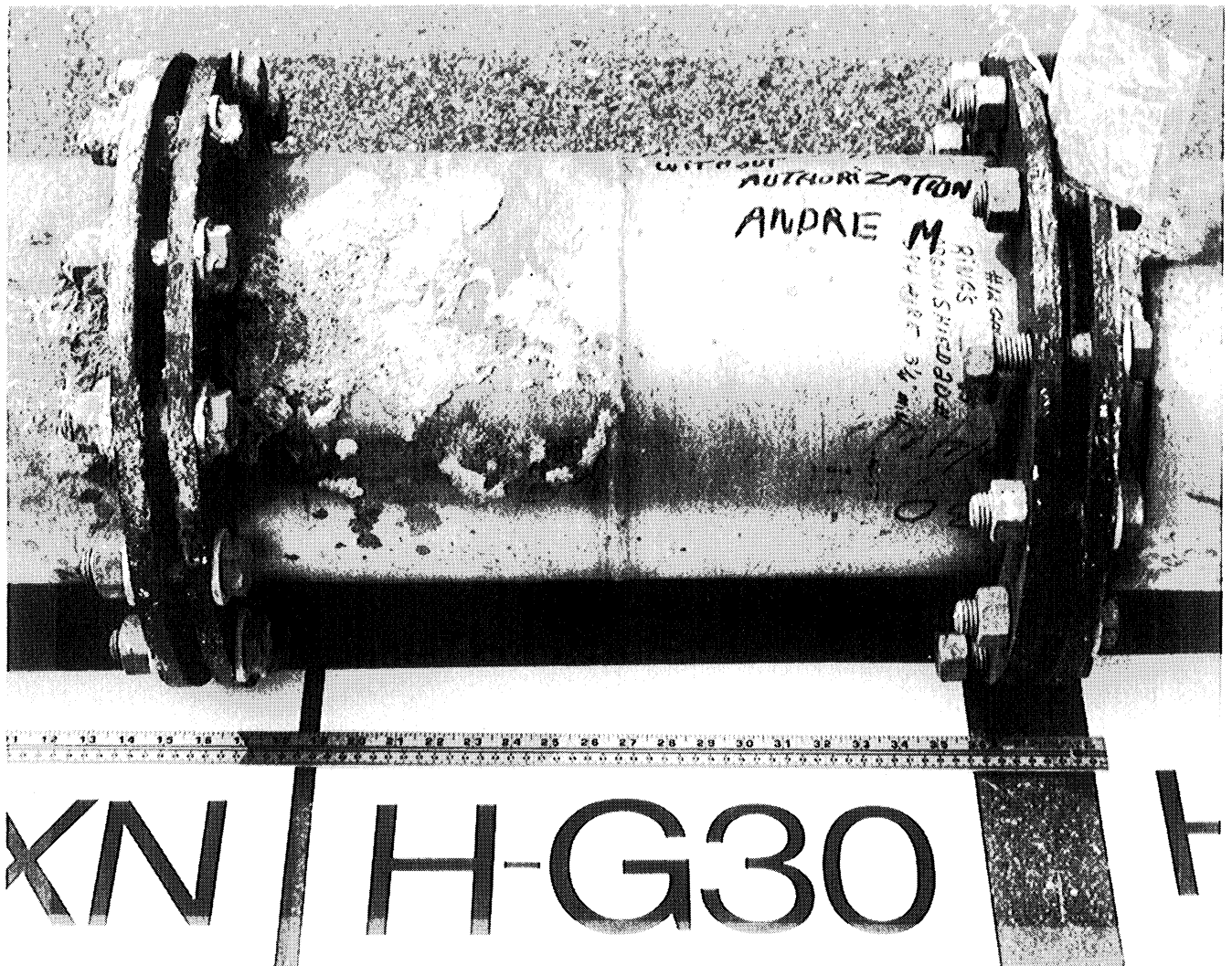
Figure 2. Typical pipe sections after chlorine dioxide filtrate service. Each section contained longitudinal and circumferential welds.
