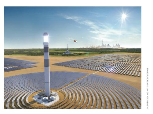
(565 °C) and a cold (290 °C) molten salt storage unit. For resistance against high temperatures and corrosion, the former is made of nickel-containing stainless steel, while the latter is made of carbon steel.
