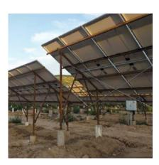
Mounting structures consist of piles for ground mounting, legs, column, beams, rail and clamps, and other assembly fixtures.
