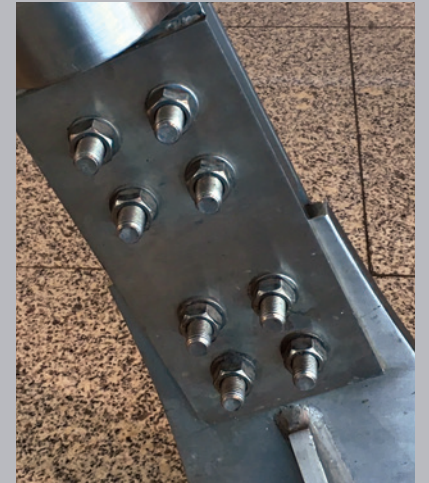
Bracing connection in a stainless steel canopy at Porto Airport, Portugal
