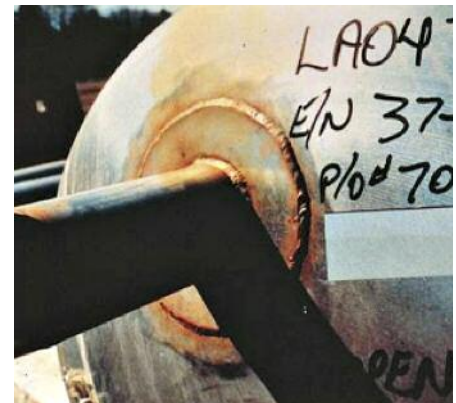
Carbon steel wire brushes used to clean stainless steel welds can produce discoloration and rust. © Outokumpu Stainless
