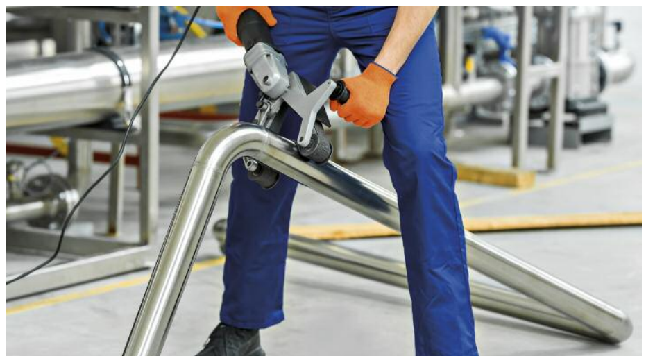
Manual polishing of a stainless steel pipe to blend the fabrication weld with the pipe surface finish. © Olya Humeniuk/Shutterstock.com
