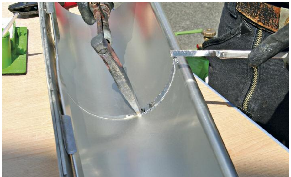
Soldering of stainless steel is not difficult, but requires a specialized flux. © BRANDT Edelstahl Dach GmbH
