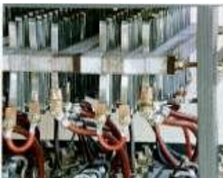
Figure 23. (DKI A 4968) Cascading Resistor with strip winding of CuNi44
