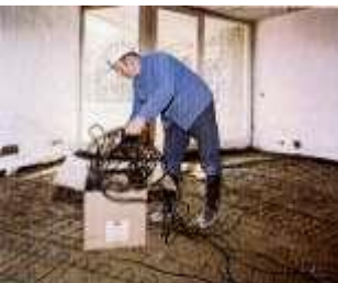
Figure 24. (DKI A 4978) Heating mat with corrugated steel sheath; resistance stranded conductor of CuNi44
