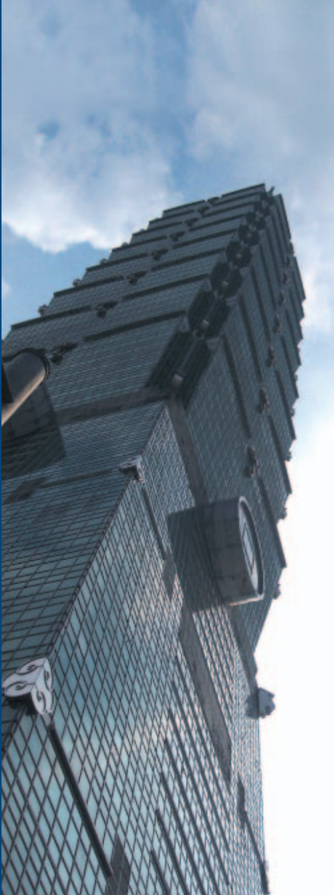
Buildings, such as the 101-storey, 509-metre-high, Taipei Financial Centre use stainless steel pipe for fire protection and hot and cold water supply.
