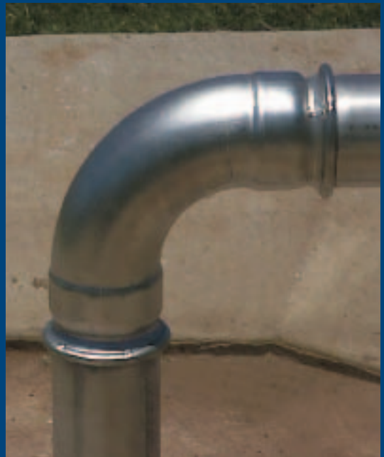
Victaulic's Pressfit joining system provides economy, reliability and fast installation.
