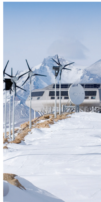
Princess Elisabeth Station, Antarctica. The façade is made of 1.50 mm 304L (S30403) stainless steel panels.
