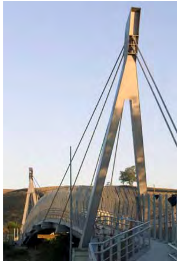
Figure 1: Pedestrian view of the completed bridge
