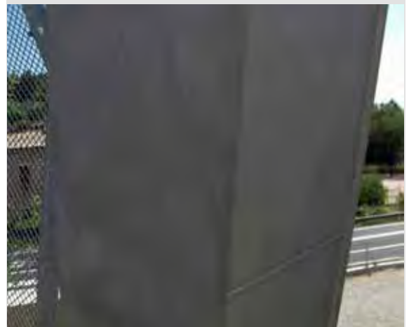
Figure 4: Welded joint on pylon
