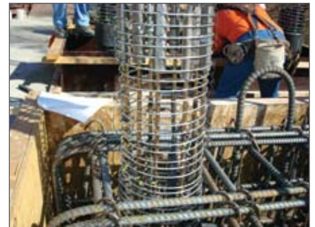
Close up of SMA bars connected to steel bars
