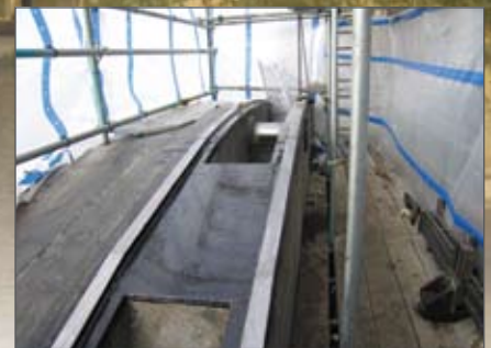
Finished rails after painting of carbon steel
