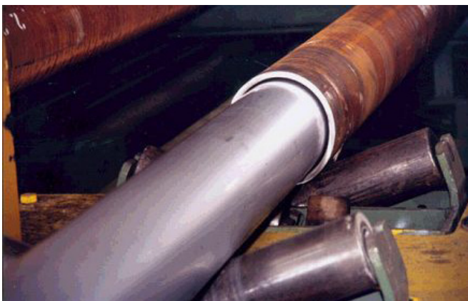
FIGURE 11. Telescopic alignment of liner and outer pipe prior to hydraulic expansion to form lined pipe.
